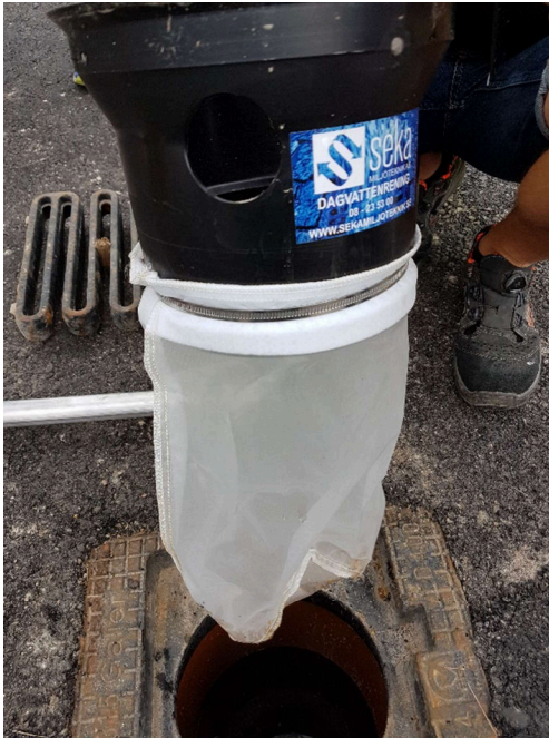
Figure 3. Granulate trap at Bergaviks IP
